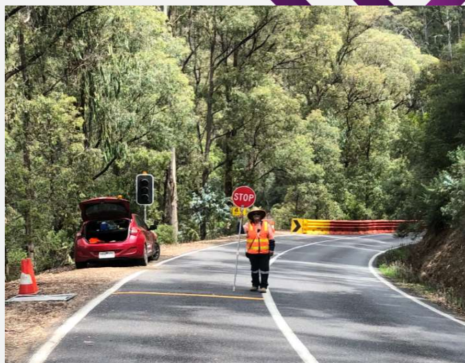
Follow the direction of roadworkers and ride safely at all times.
